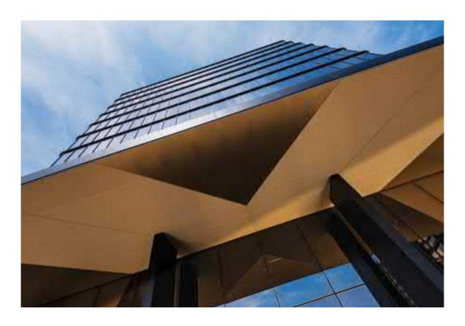
The building consists of one building, located in Viale Sarca at No. 235. The project led to the redevelopment of the building, its basement car park and the related external arrangements. The renovation project has enhanced the features of the existing building; the existing curtain wall system was replaced with a new façade that is transparent, modular, simple and with a clear shape.
