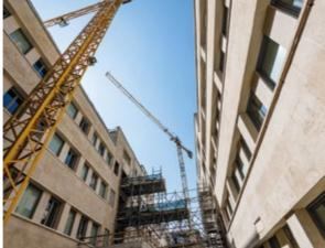
For this project, Carron acts both as promoter and builder of nursing homes in Turin. After purchasing two symmetrical buildings, Carron is completing their renovation through the complete demolition and removal of all the walls, as well as structural reinforcement works, the remake of all the internal finishes and the implementation of new installations. The functional recovery of the buildings will lead to two separate nursing homes with 200 beds each, both subject to sales as future assets.
