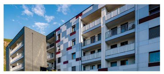
Energetic renovation of 72 apartments that remain inhabited during the works, renovation works in compliance with the "CasaClima A" regulations, new façade with prefabricated wooden panels, mixed heating and DHW system: geothermal heat pump + integration with boiler, solar photovoltaic plus solar thermal, mechanical ventilation with decentralised system for each apartment.
