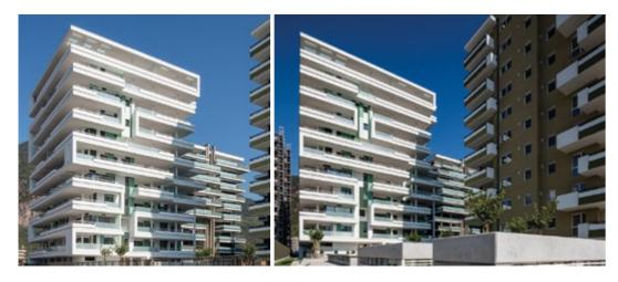
This new construction complies with the "CasaClima NATURE" regulations with high hygiene standards and a careful management of waste. The building height equals to 34 metres with 11 aboveground floors, the work site is surrounded by other lots implemented simultaneously (not part of our job order), two large floors underground with 0-height waterproof slabs (Zementol system).
